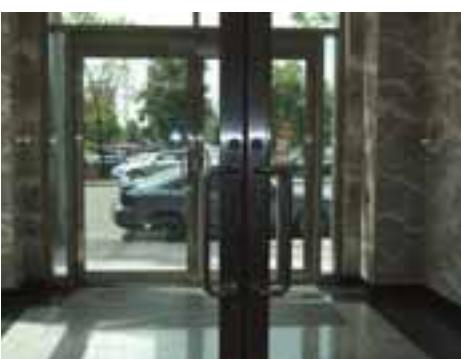
Here is a set of double doors. Even though the handles are clearly labelled with the words "Push," since you can grip the handles, a number of people will try to pull them. Solution: remove the handles and attach a flat panel to make it obvious that the door is to be pushed.
